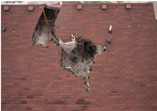
Helicopter enters the home from the back
