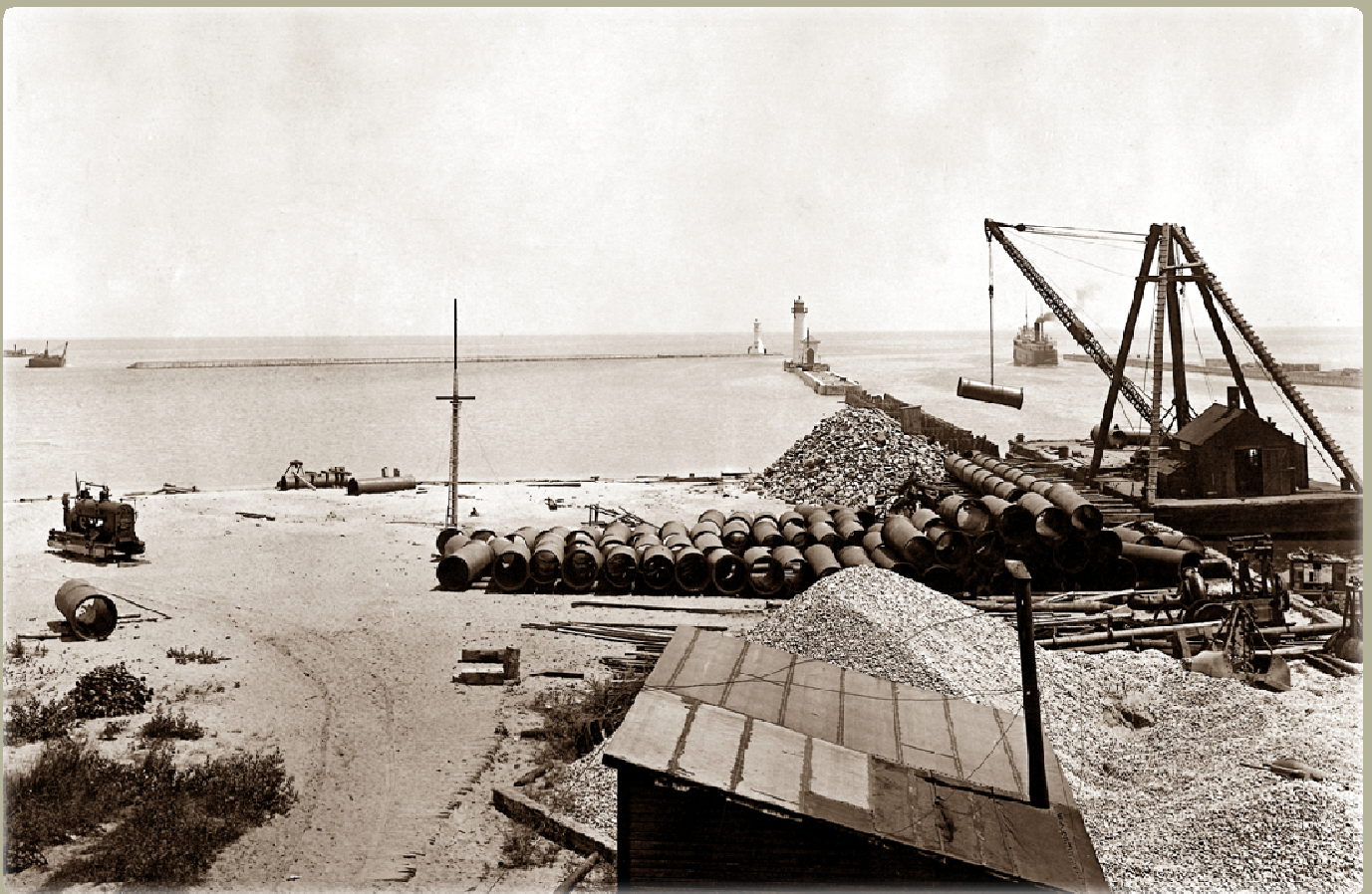
Installation of 42" intake pipe - 1916
