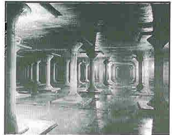
Inside 2.5 Million Gallon Finished Water Reservoir - 1926
