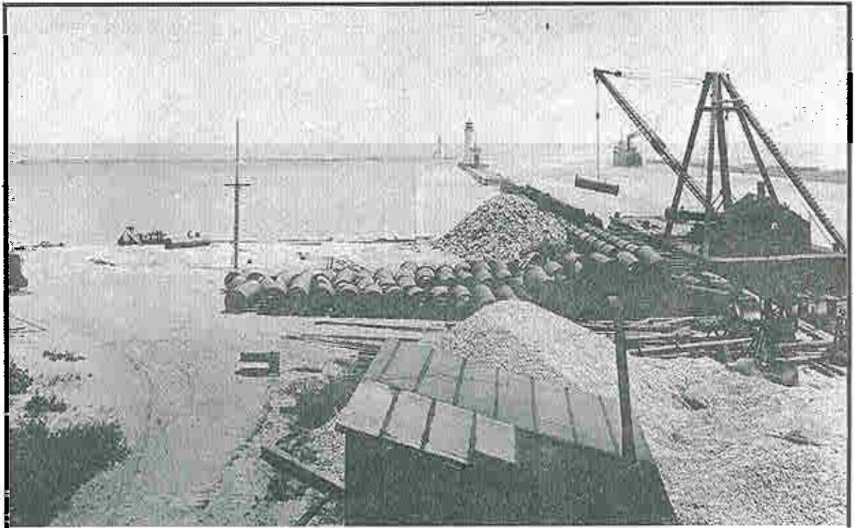
Installation of 42" Cast Iron Intake Pipe into Lake Michigan - 1916
