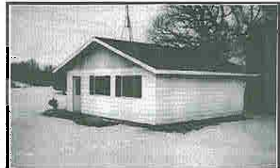
New booster station at 7th Avenue & 80th Street - 1988
