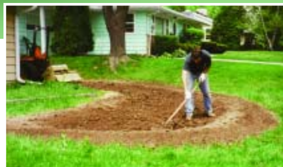
On a gentle slope, soil from digging out the garden can be used to create the berm. This rain garden is 4 inches deep.
