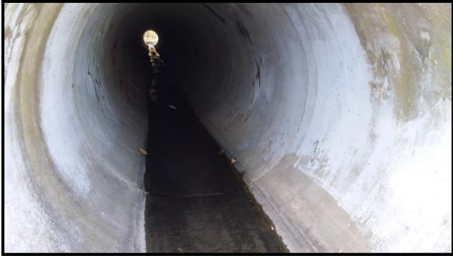
Image 1 Stormwater Sewer in Jamestown Park. 2019
