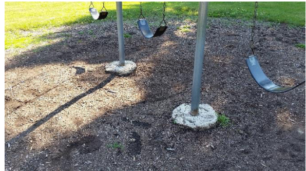
Exposed footings in fall zones of swings
