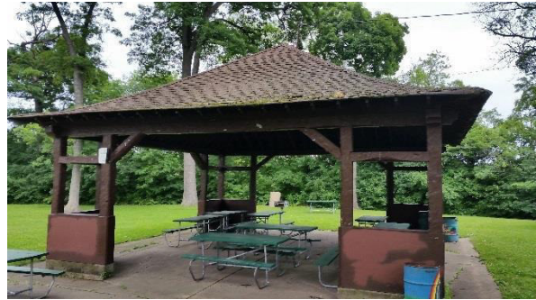
Small shelter (Area 1)
