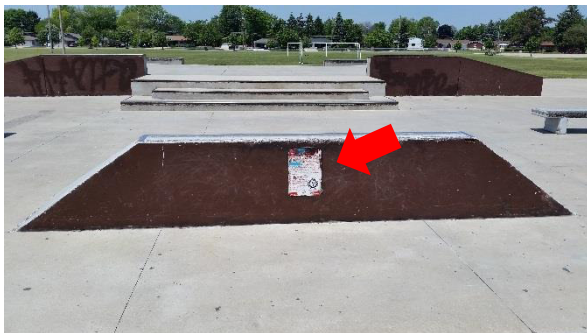
Poorly placed rules sign
