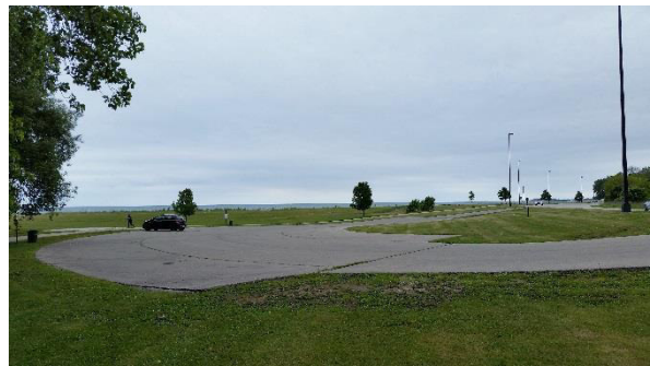
Parking lot (Area 2)
