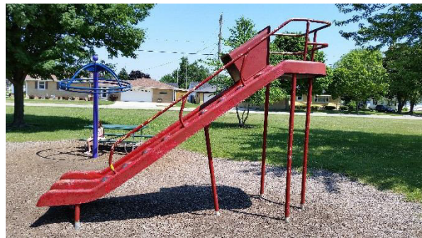
Slide in poor condition - REMOVED
