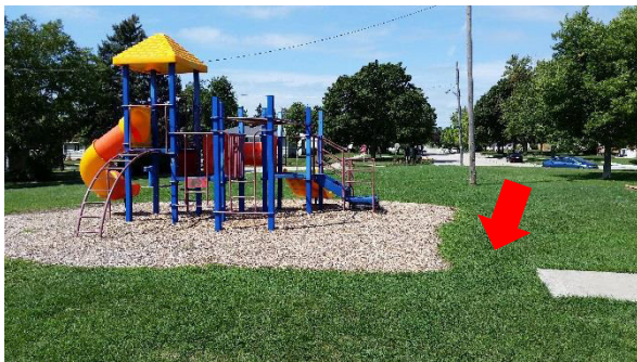
No ADA access to facilities
