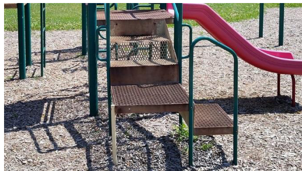
Play structure steps are worn
