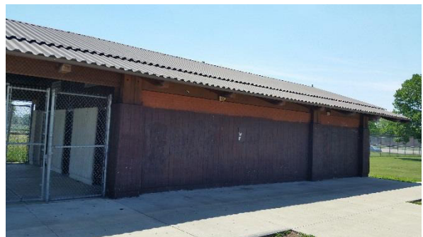
Restroom building under contract to be removed
