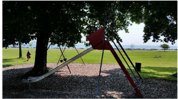
Tree encroaching on play equipment
