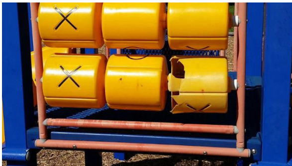
Play structure damage
