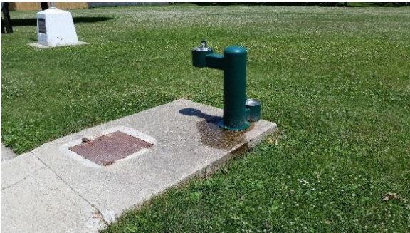
Drinking fountain access issues
