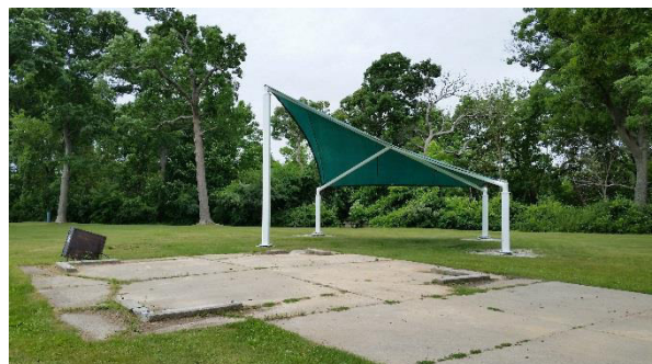
Shade structure & former shelter pad (Area 3)
