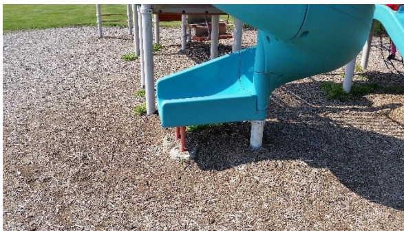
No safety mats under play equipment
