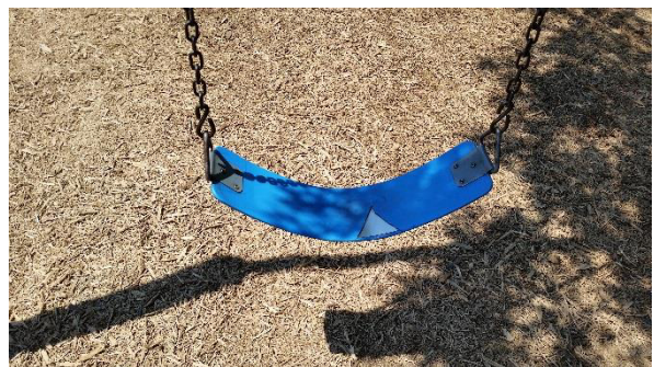
Swing seat in poor condition
