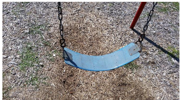
Swing seat in poor condition
