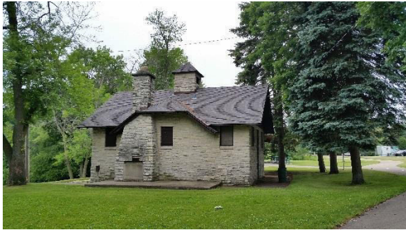
Restroom building (Area 1)
