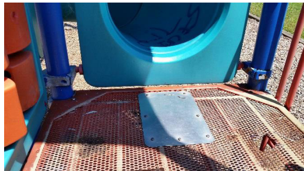
Play structure in poor condition
