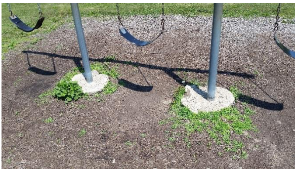
Exposed concrete footing in swing fall zones
