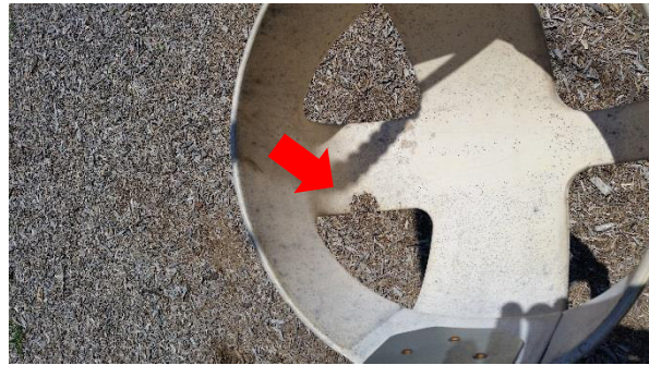
Bucket swing seats are damaged
