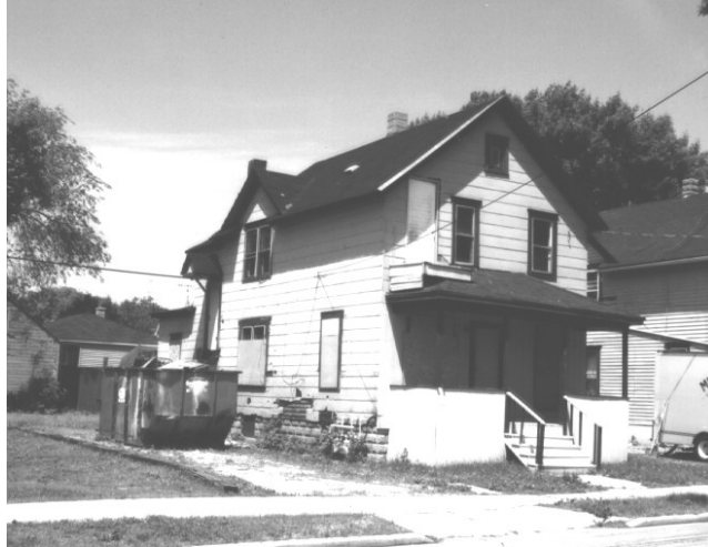
An example of the most substandard or deteriorated house in the Lincoln Neighborhood.
