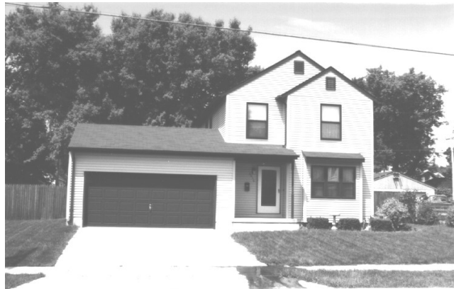
The most recently constructed single-family infill houses resemble a typical two-story suburban ranch with a 2-car attached garage.
