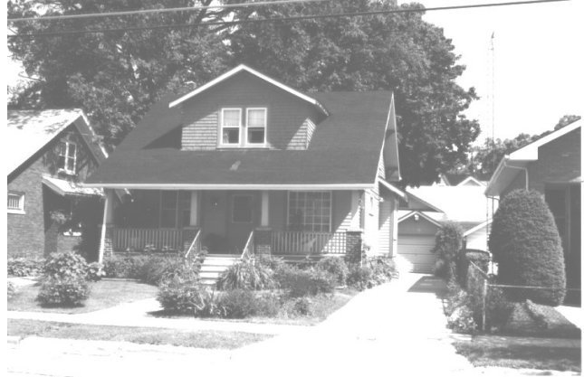
Porches are generally located under the main roof and extend the full width of the house.
