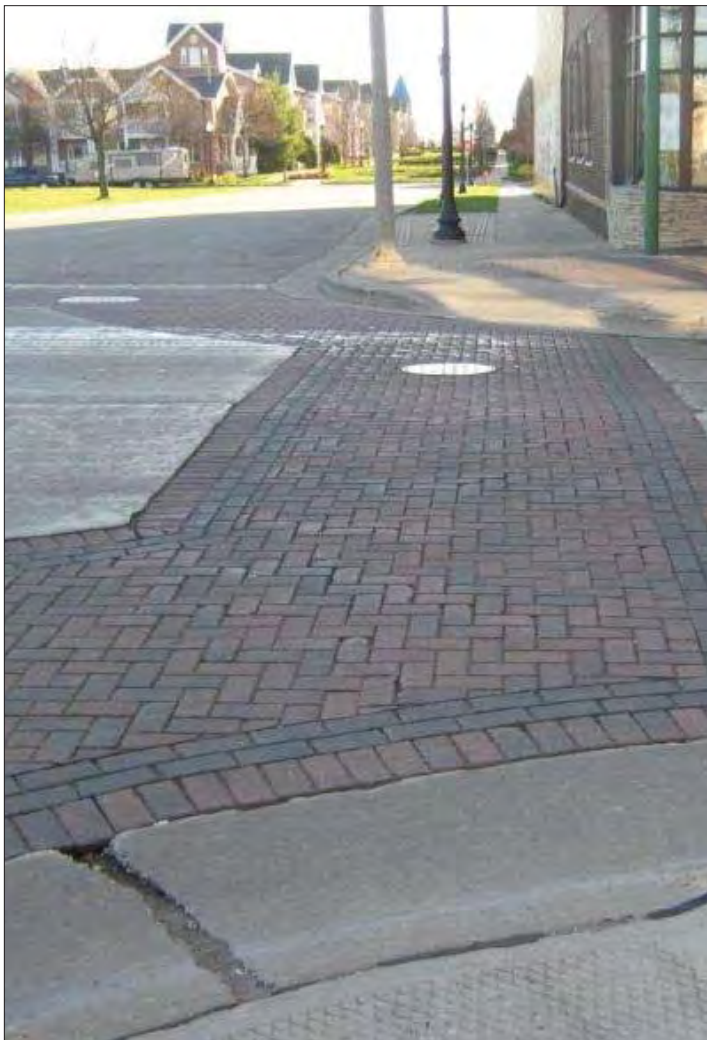
White crosswalk markings would provide better visual notifications alerting drivers to watch out for pedestrians.
