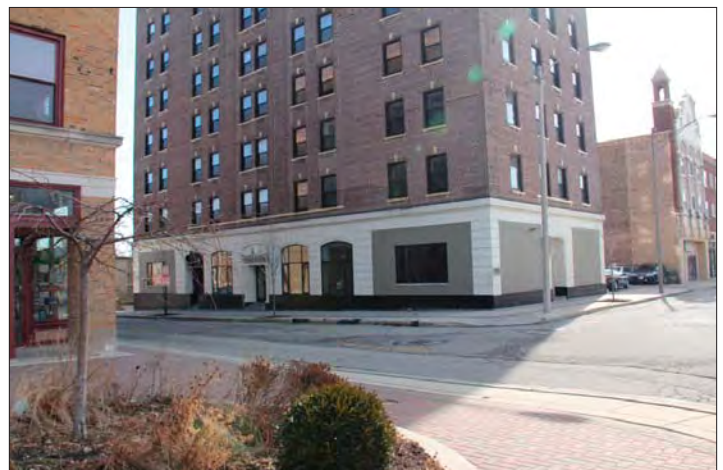
Dayton Residential Care Facility at street level
