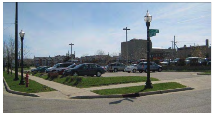
Existing curb ramps are constructed with a diagonal ramp. Where possible, one ramp should be provided for each crosswalk, and crosswalk markings should be added.
