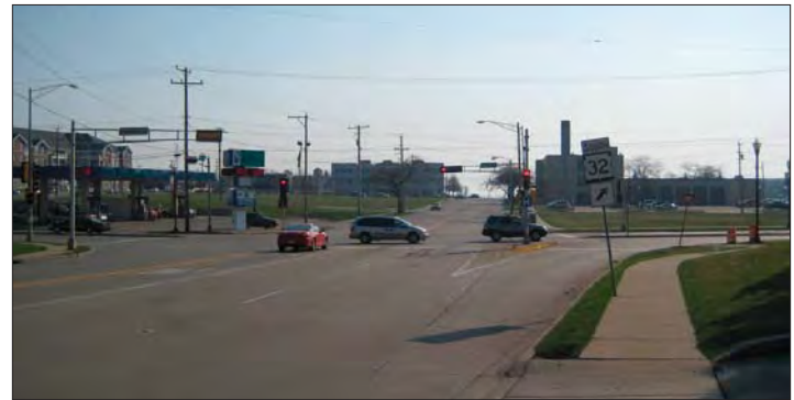
Eastbound 52nd Street (STH 158) is the only main roadway from I-90 that goes to the lakefront. At Sheridan Road, 52nd Street fails to visually draw you into Downtown.
