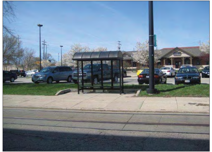
A waiting shelter for the streetcar is provided at the Metra Station. Streetcar signage (on the street light pole) is small and mounted too high to be easily seen.
