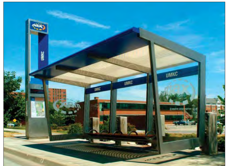
A new, covered bus stop in Kansas City, Missouri.
