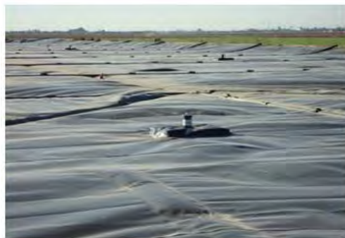
Covered Lagoon Digester
